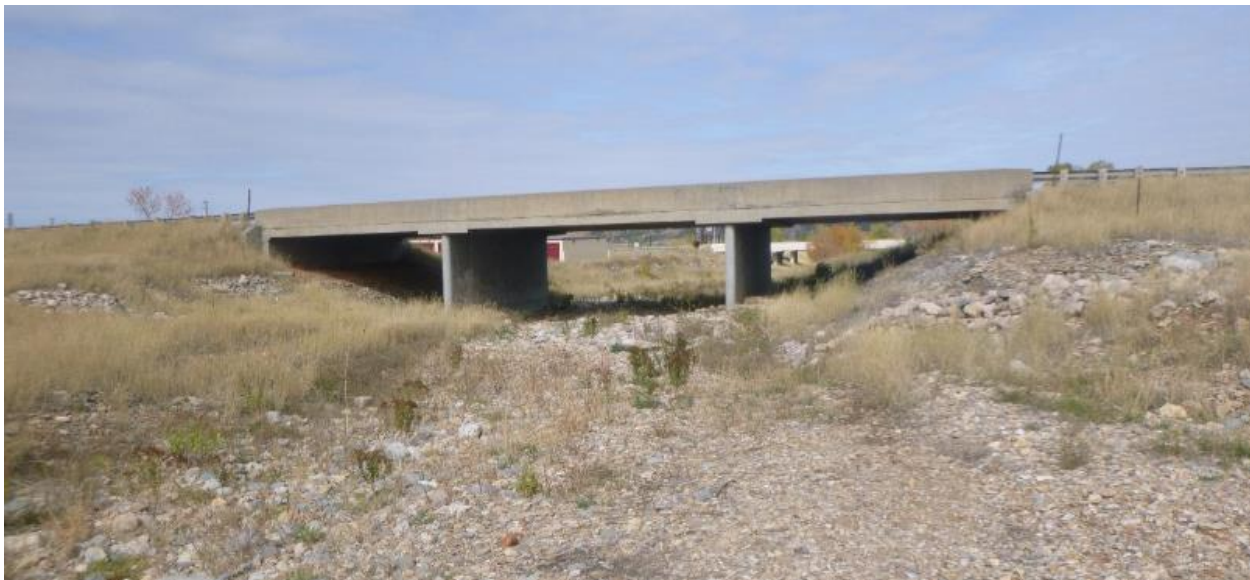
Figure 13. False Bottom Creek Bridge – South Elevation Looking North
