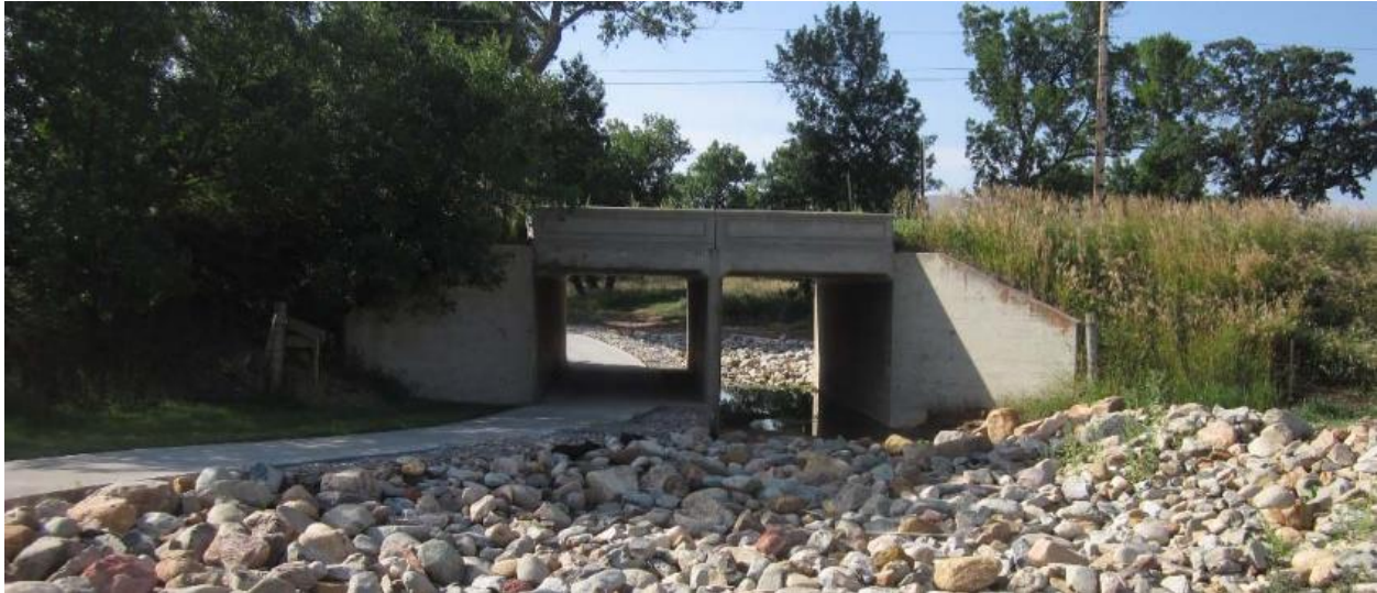
Figure 14. Miller Creek Box Culvert – South Elevation Looking North
